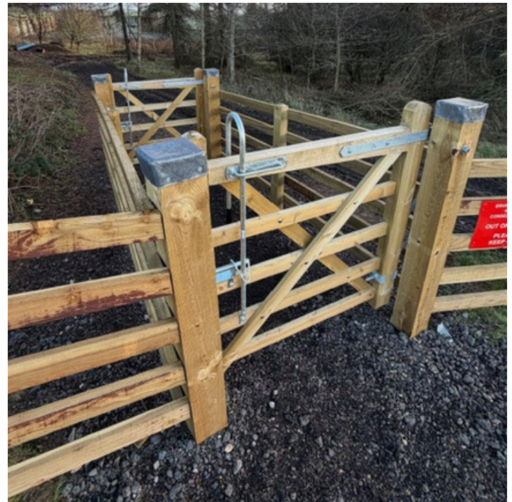
Gate at the new entrance to Foxglove Covert.
